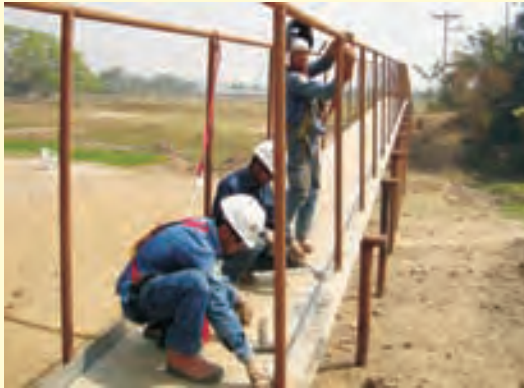
In linking the two banks of the Norkhai River, the Chevron-constructed Bibiyana Friendship Bridge served about 15,000 to 20,000 residents. Connecting the villages of Karimpur and Chanpur, the 160-foot (predominantly steel) footbridge provided the local community safe and easy passage, particularly during the rainy season.
