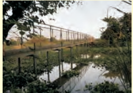
In linking the two banks of the Norkhai River, the Chevron-constructed Bibiyana Friendship Bridge served about 15,000 to 20,000 residents. Connecting the villages of Karimpur and Chanpur, the 160-foot (predominantly steel) footbridge provided the local community safe and easy passage, particularly during the rainy season.
