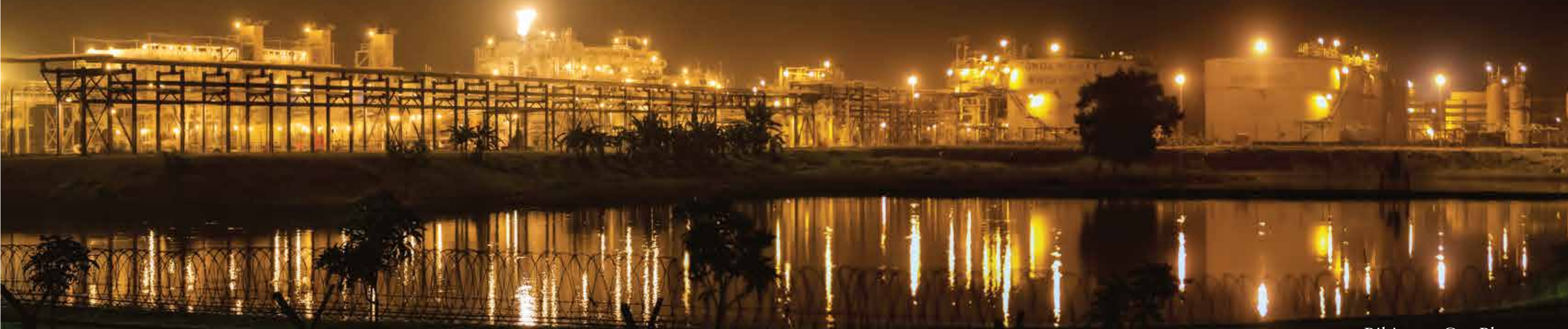
Bibiyana Gas Plant
